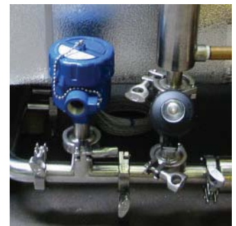
Water Sensor in Drain/EN285 Air Detect Assembly
